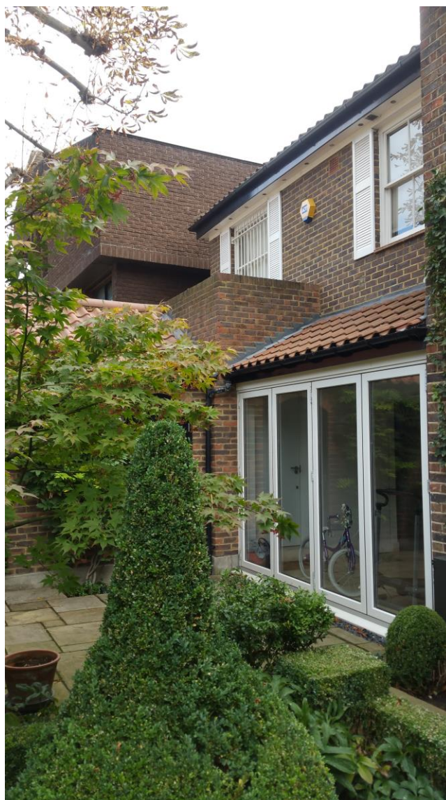
North West elevation facing Elm Tree Road, with neighbouring property at No. 4A Elm Tree Road in background.
