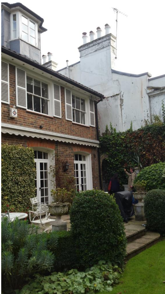
South West elevation facing Grove End Road, adjoining No. 14 Grove End Road
